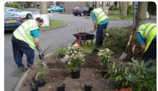
Quadron team preparing planting beds at Anstice Close
